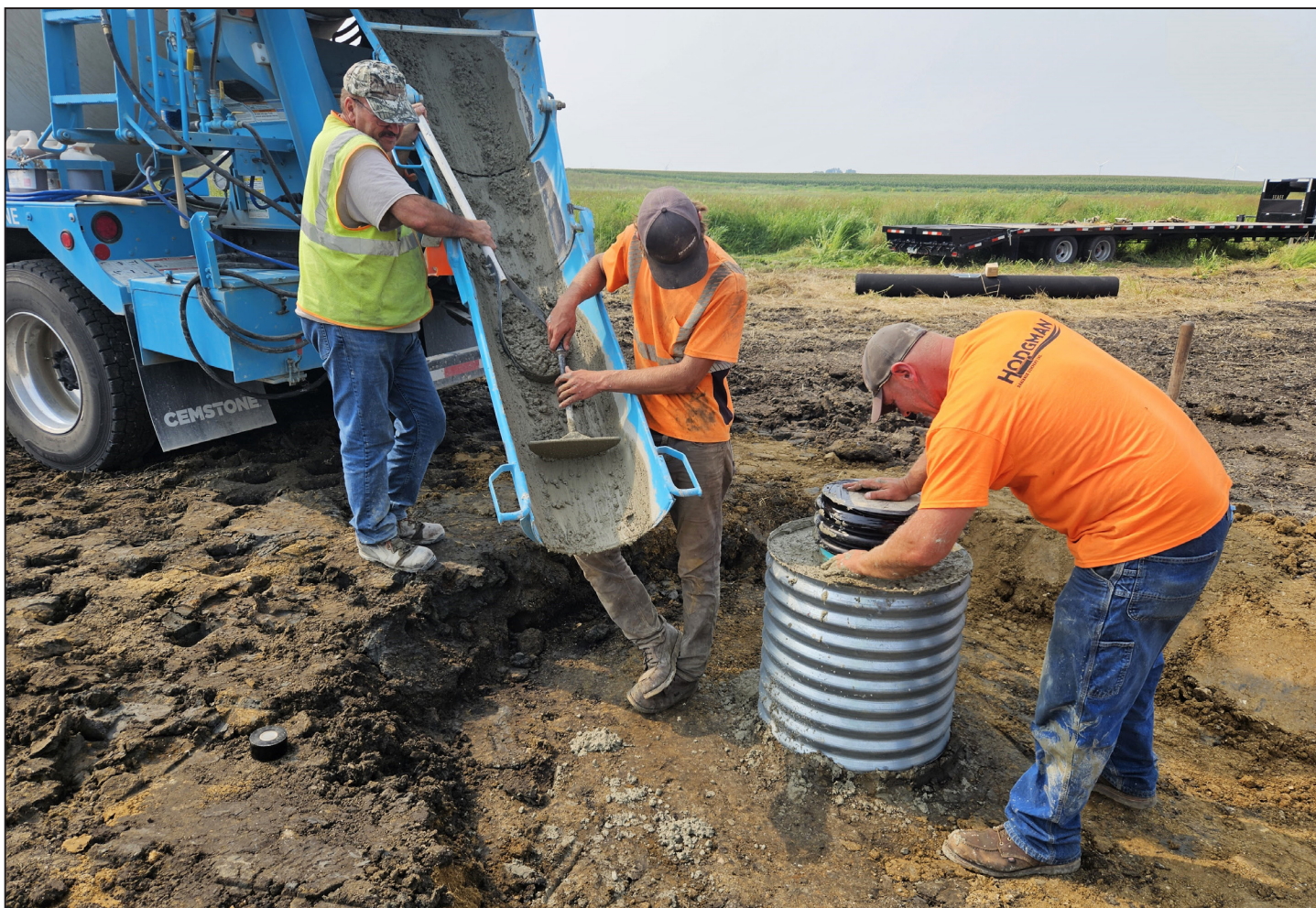
Workers from Dodge Center-based Hodgman Drainage Co. constructed the primary outlet structure for the wetland restoration in August. Structures like this one help control water flow, regulating the quantity and speed of water as it is released from a wetland.
