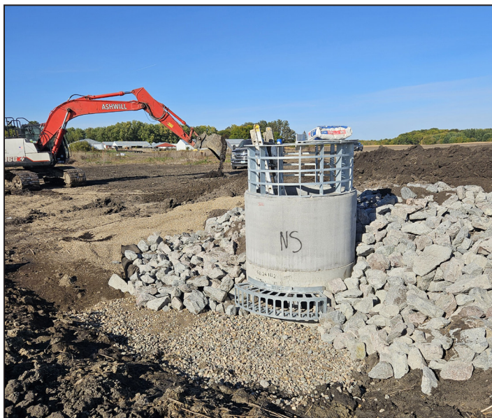
An outlet structure was installed as part of the wetland restoration work. Construction began in July 2024 and concluded in October.
