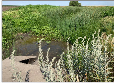
Left and right: Phase 2 of the Whiskey Creek stream restoration, seen here on Aug. 2, 2022, connected to Phase 1 work completed in fall 2021, which created 4.3 remeandered stream miles within a 3.3-mile corridor along Minnesota Highway 9 in central Wilkin County. Middle: Vegetation flourished along a segment of Whiskey Creek. Remeandering the once-straightened channel will help to slow velocity, curb bank erosion and avoid sediment build-up.
