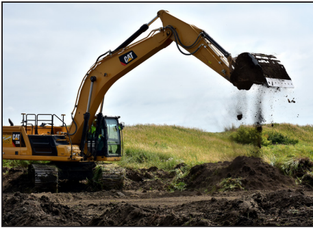
Left and right: Phase 2 of the Whiskey Creek stream restoration, seen here on Aug. 2, 2022, connected to Phase 1 work completed in fall 2021, which created 4.3 remeandered stream miles within a 3.3-mile corridor along Minnesota Highway 9 in central Wilkin County. Middle: Vegetation flourished along a segment of Whiskey Creek. Remeandering the once-straightened channel will help to slow velocity, curb bank erosion and avoid sediment build-up.
