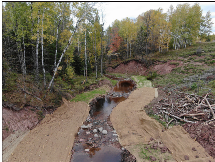
Top: A stream restoration on a 500-foot length of Stateline Creek used natural channel design methods to narrow and stabilize the channel, and to re-establish connection to the natural floodplain. A series of constructed riffle pools allow fish passage. The project also addressed streambank erosion. Bottom: This post-construction view of Stateline Creek was captured in 2021. Photo Credits: Carlton SWCD
