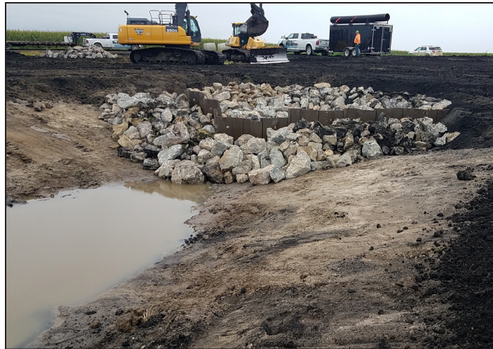
Construction was completed by Byron-based DeCook Excavating in 2020 and includes three large shallow wetland pools, an inlet structure (above) and an outlet structure (below).
