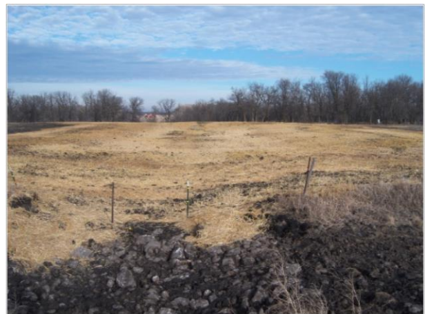
Grassed waterway and drop structure completed in 2012.
