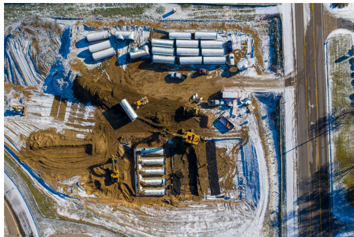
Above: Stormwater from a 46-acre watershed drains to the Ramsey County Road B storm sewer adjacent to Parkview Center School in Roseville. Now cleaned water treated at the site discharges through the storm sewer and runs through wetlands at Villa Park before entering Lake McCarrons. Below: Original plans called for siting the project under school athletic fields. But groundwater was too close to the surface there, so it was worked into a hillside.
