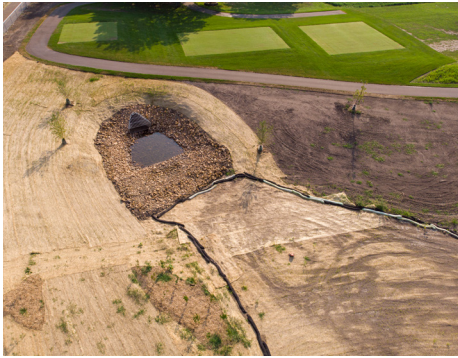
Previously untreated runoff from 612 acres now flows from east to west through Columbia Golf Course and Columbia Park, where it is diverted to a treatment pond, a dry basin, and then an infiltration basin before it re-enters the stormwater sewer system and continues on for 1.2 miles to the Mississippi River. The Clean Water Fund-supported project is slated to wrap up this month. Photo Credits: Mississippi WMO
