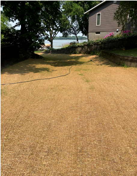
AFTER: The completed project, seen here on July 21, 2021, incorporated new tile and a regraded slope covered by erosion control fabric made of jute. It will keep an estimated 2.1 tons of sediment and 2.1 pounds of phosphorus out of Circle Lake each year.
