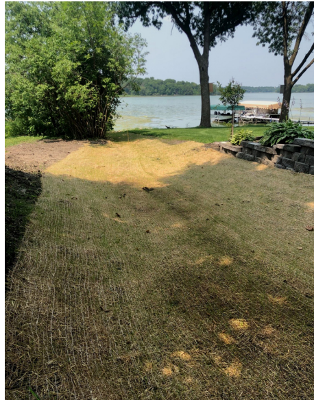
AFTER: The completed project, seen here on July 21, 2021, incorporated new tile and a regraded slope covered by erosion control fabric made of jute. It will keep an estimated 2.1 tons of sediment and 2.1 pounds of phosphorus out of Circle Lake each year.
