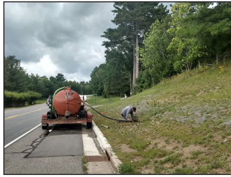
Left: Inlets to underground sediment collectors lie just off Crow Wing County Road 66 at Big Trout Lake. Middle: Maintenance involves periodic removal of accumulated sediment. Right: Crow Wing SWCD Manager Melissa Barrick posed with AmeriCorps intern Reece Boucher in 2018 along Big Trout Lake where a sediment collector was to be installed. Photos Courtesy of Crow Wing SWCD
