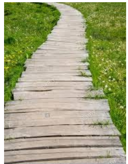
Non-elevated walkway (fill)
