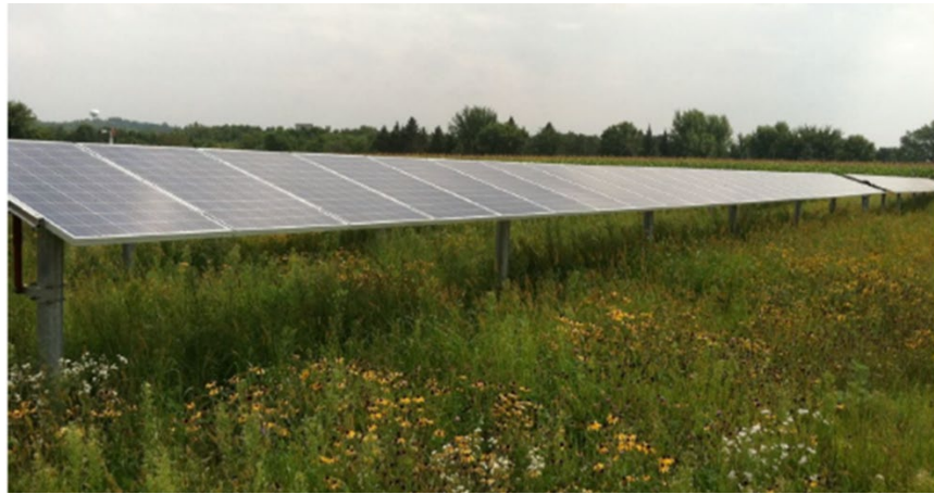
Pollinator-friendly plantings under and around solar panels.
