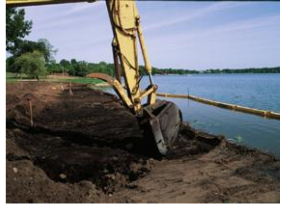
The removal of fill as part of a shoreline restoration project
