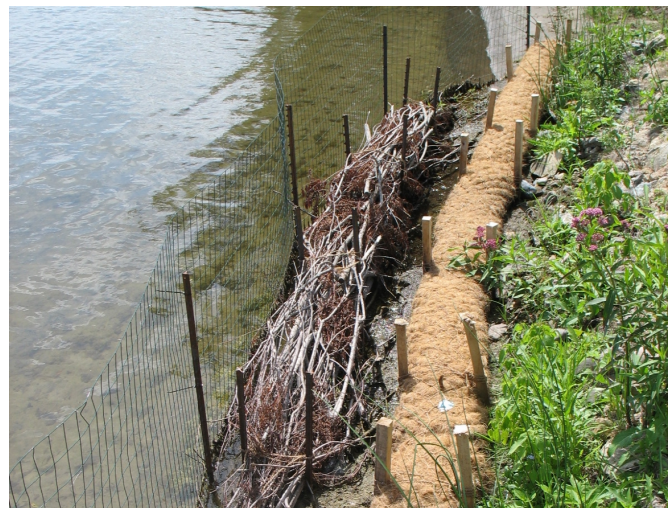
Shoreline restoration using wood mulch, coconut fiber bio-logs, wattles and fencing
