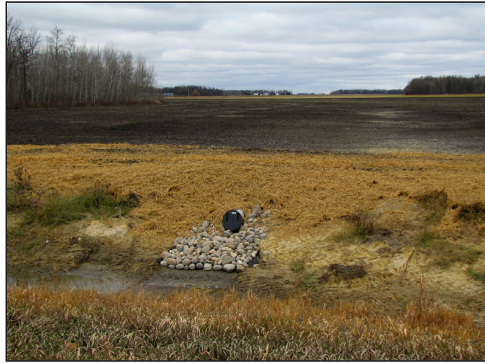
While not in a prioritized subwatershed, this Pennington County site is an example of a side-water inlet. Photo Credit: Pennington SWCD
