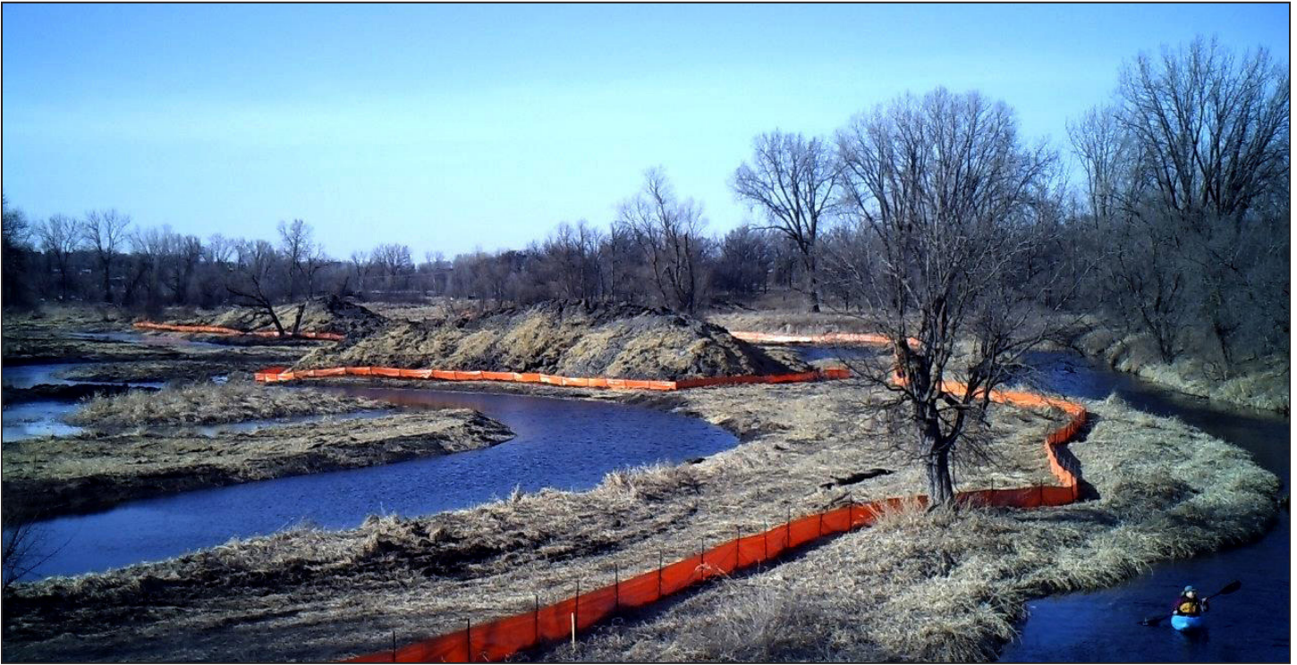
A Rice Creek Watershed District trail camera captured paddlers using the original, previously straightened stream while the remeandered segment of Middle Rice Creek, at left, was being constructed. Photo Courtesy Rice Creek Watershed District
