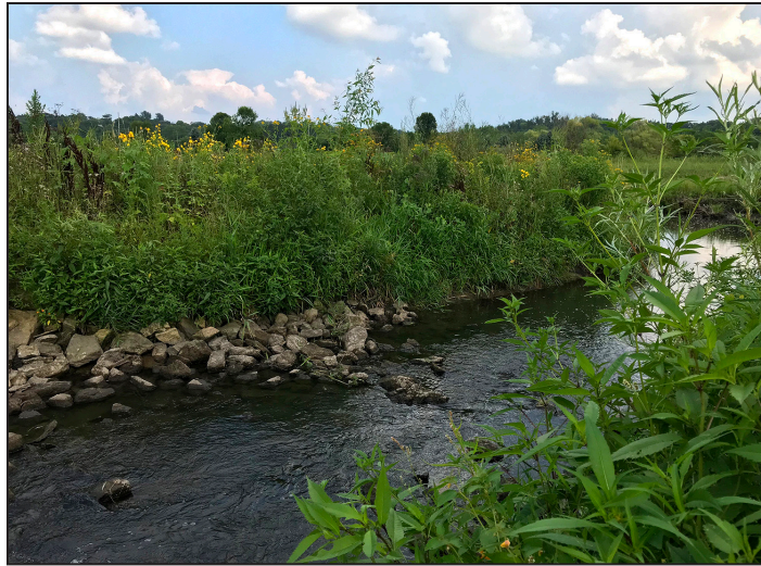
The redesigned South Branch of Cascade Creek mimicked the sinuosity, dimension and shape of a stable channel elsewhere in the watershed.
