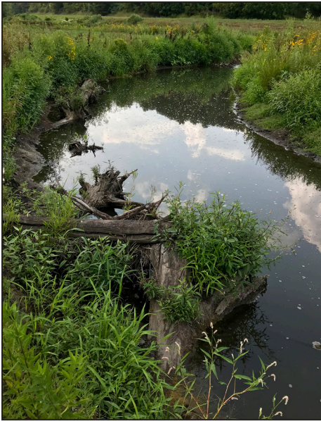
Left: Root wads help to stabilize the banks of the South Branch of Cascade Creek. Middle: Rocks were placed to slow the water, create habitat and stabilize the streambed of the South Branch of Cascade Creek. Curves were designed to help curb the velocity. Right: Wetlands eventually will fill with water. Logs and roots will help to create habitat. Engineers hope the wetlands will distract beavers and keep them from damming the creek.
