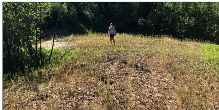
Melanie Bomier, Carlton Soil & Water Conservation District water resources technician, puts into perspective the size of a project that replaced a failed red clay dam.
