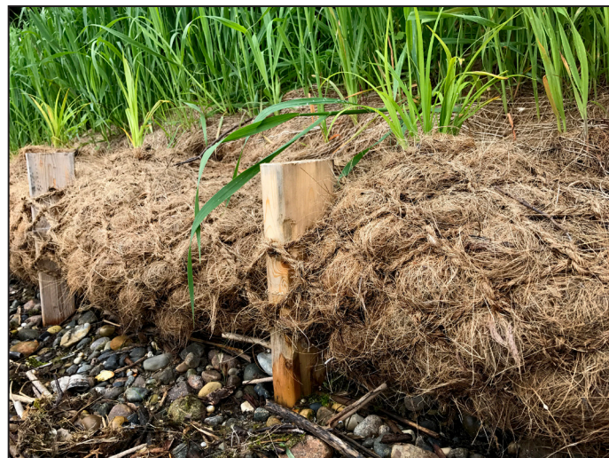
BELOW: Hemp rope and coconut-fiber matting anchor a shoreline restoration on Detroit Lake. They will decompose over time, as will the wooden stakes. While a true restoration would bring back trees, the SWCD is balancing landowners' desire to use their property for recreation with what's best for the lake and for wildlife.
