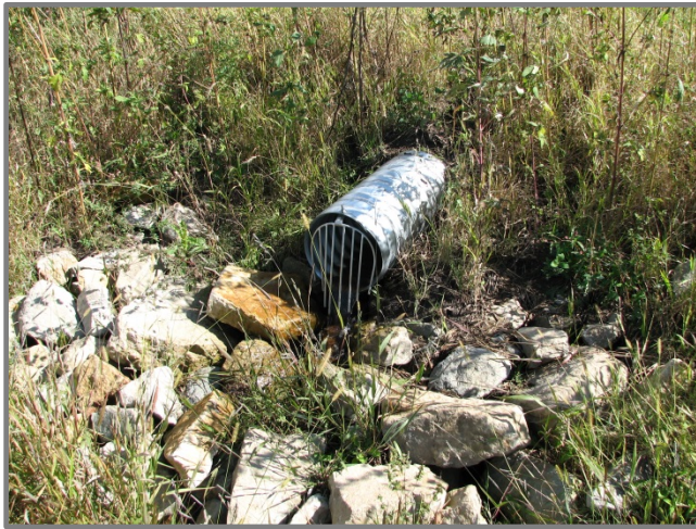
Figure 6. Riprap Protection at Tile Outlet
