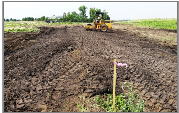
Figure 11. Compaction of Constructed Ditch Plug
