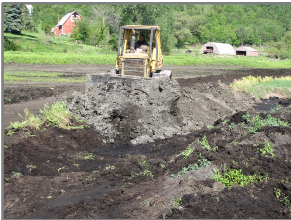
Figure 2. Shallow Ditch Being Filled
