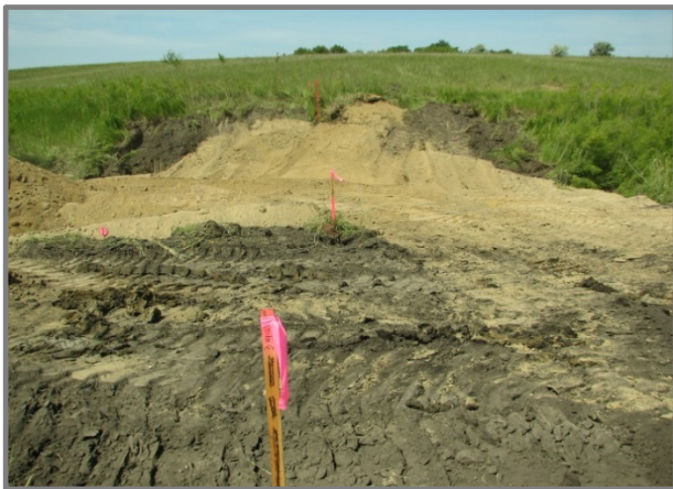
Figure 10. Ditch Plug under Construction
