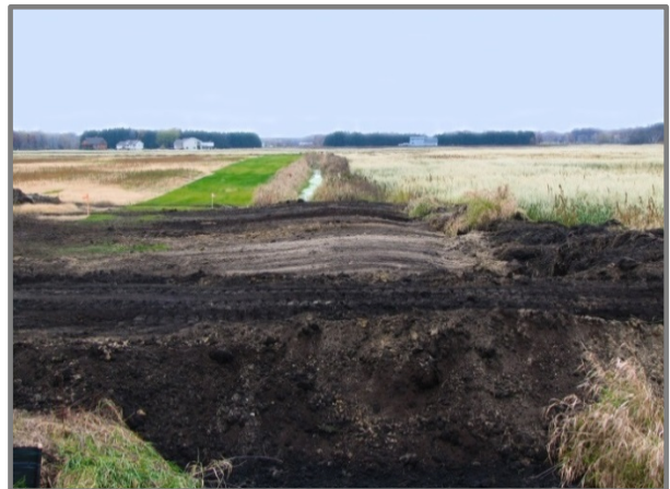
Figure 12. Finished Ditch Plug with Crown in Middle
