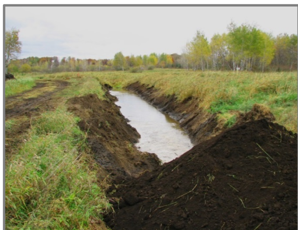
Figure 7. Importing Material to Fill Ditch thru Non-Depressional Wetland
