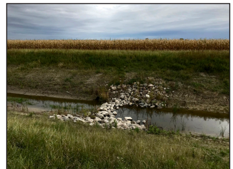
Left: Gently sloped sides are one element of a Traverse County Ditch 37 retrofit. The retrofit will help alleviate flooding in farm fields and improve water quality within the Bois de Sioux Watershed by allowing nutrient-carrying sediment to settle. Middle: Side-inlet culverts in the berm connect the ditch to the field. When the water level in the ditch is high, the pressure pushes a flap-gate shut. Water then remains on the field until the level in the ditch drops. Right: Check dams help to reduce the velocity within the ditch.
