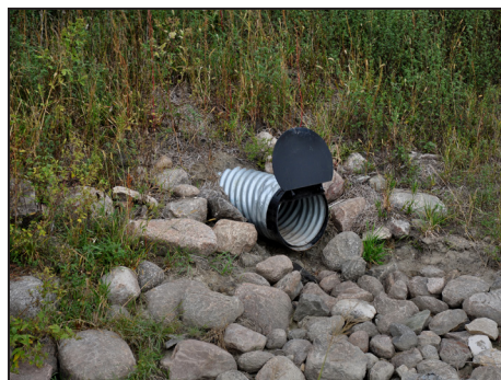
Left: Gently sloped sides are one element of a Traverse County Ditch 37 retrofit. The retrofit will help alleviate flooding in farm fields and improve water quality within the Bois de Sioux Watershed by allowing nutrient-carrying sediment to settle. Middle: Side-inlet culverts in the berm connect the ditch to the field. When the water level in the ditch is high, the pressure pushes a flap-gate shut. Water then remains on the field until the level in the ditch drops. Right: Check dams help to reduce the velocity within the ditch.
