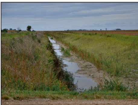
Left: Gently sloped sides are one element of a Traverse County Ditch 37 retrofit. The retrofit will help alleviate flooding in farm fields and improve water quality within the Bois de Sioux Watershed by allowing nutrient-carrying sediment to settle. Middle: Side-inlet culverts in the berm connect the ditch to the field. When the water level in the ditch is high, the pressure pushes a flap-gate shut. Water then remains on the field until the level in the ditch drops. Right: Check dams help to reduce the velocity within the ditch.
