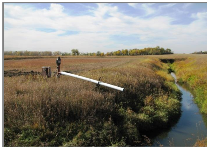
Figure 1. Tile Drained Wetland Aided by Lift Station
